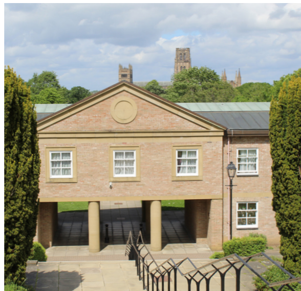
The Williamson building, built in 1962
